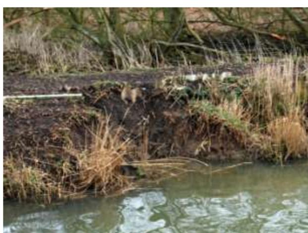
*Significant damage to New Cut by deer. Exposed asbestos sheeting along bank of New Cut*
